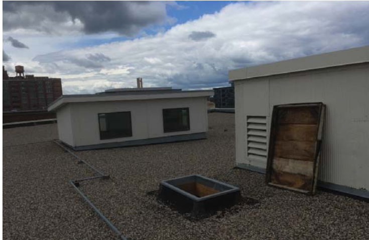
Existing Roof Condition
