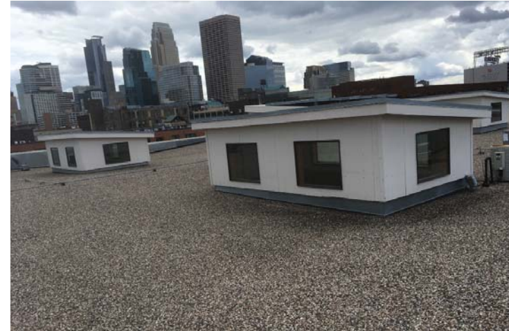
Existing Roof Condition
