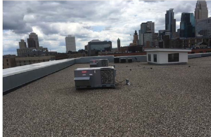
Parapet on Washington Avenue
