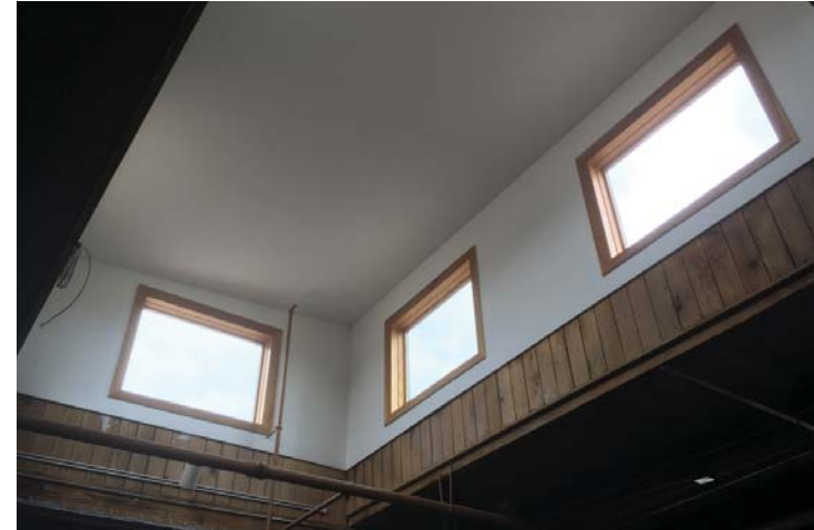
Existing Interior Conditions
